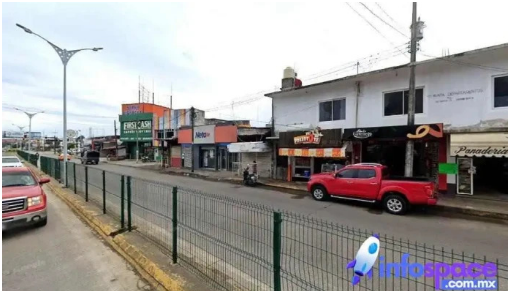
Terminal transportes san jose chiltepec san juan bautista tuxtepec
